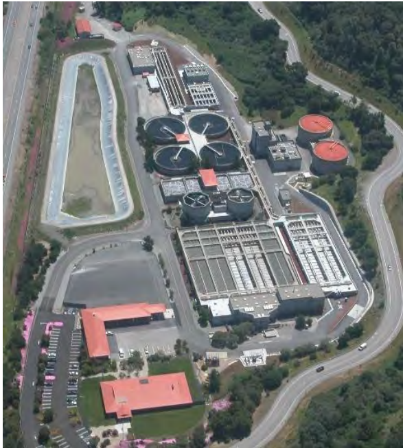
Photo provided courtesy of CMSA
