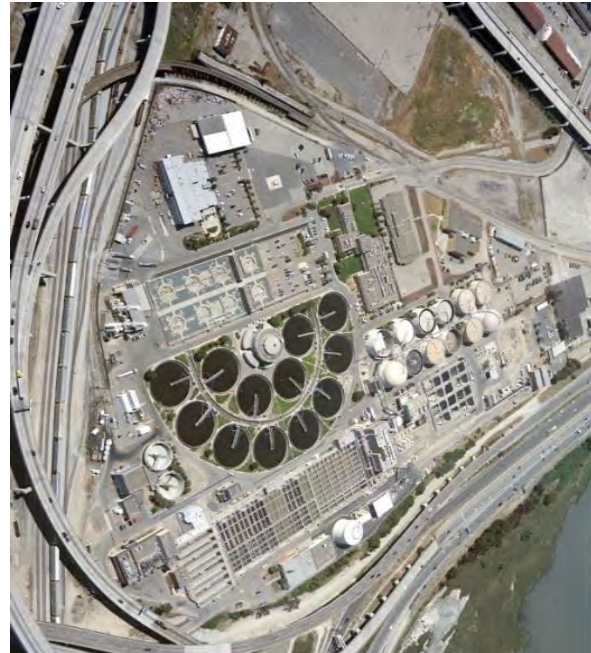
Photo provided courtesy of EBMUD
